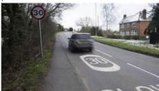
Speed roundels are road markings which give motorists a clear indication of the road speed limits and have help slow traffic speed.
